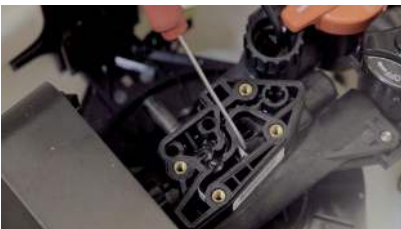
Replacement of internal valve components
