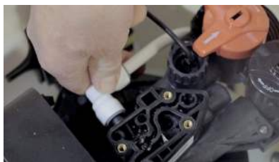
Replacement of brine delivery elbows
